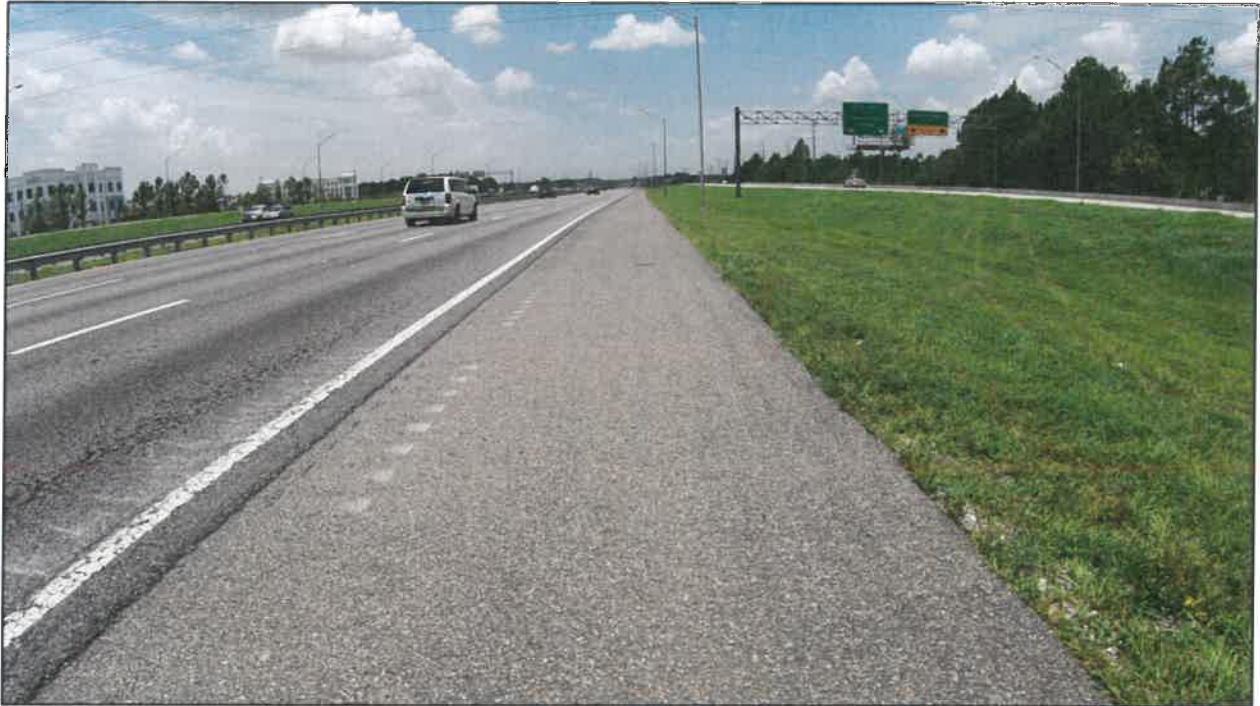
Photo 12: I-4 westbound near MP 4.960. This is a location where limerock pumping was observed in the outside wheelpath of the L3 lane. This is a lane that was widened in 2006, not the original alignment.
