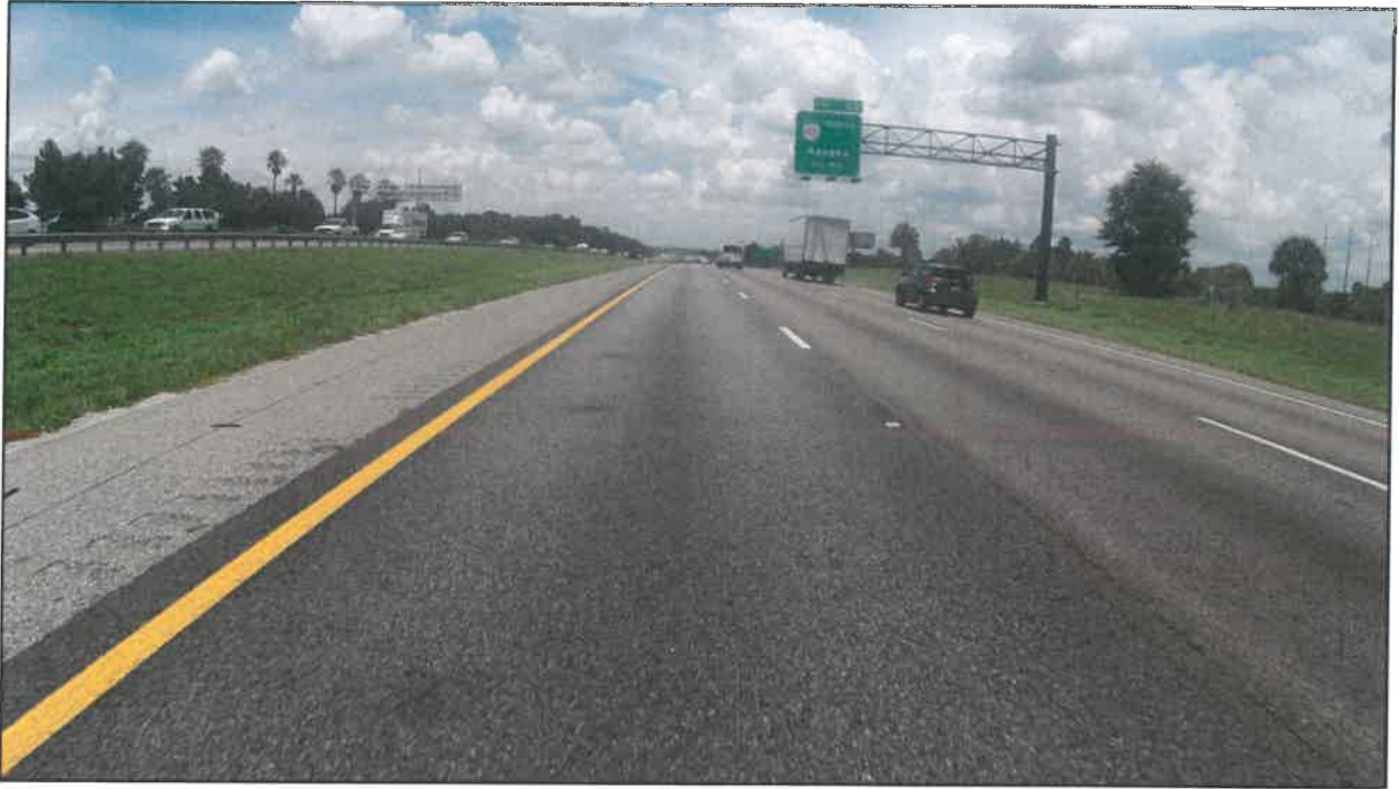
Photo 1: I-4 eastbound near MP 0.741. This picture shows the typical fair condition of the R1 inside passing lane within the project limits.
