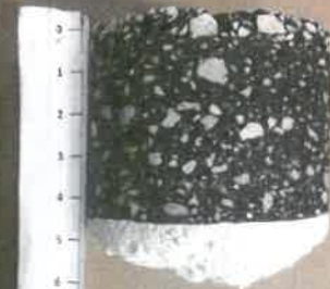
Core #107 500' West of bridge over Bonnet Creek on I-4 EB to Osceola Pkwy, RAMP
