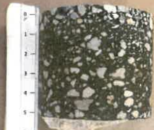
Core #95 500' West of Bridge over Bonnet Creek on I-4 WB to Osceola Pkwy WB, RAMP
