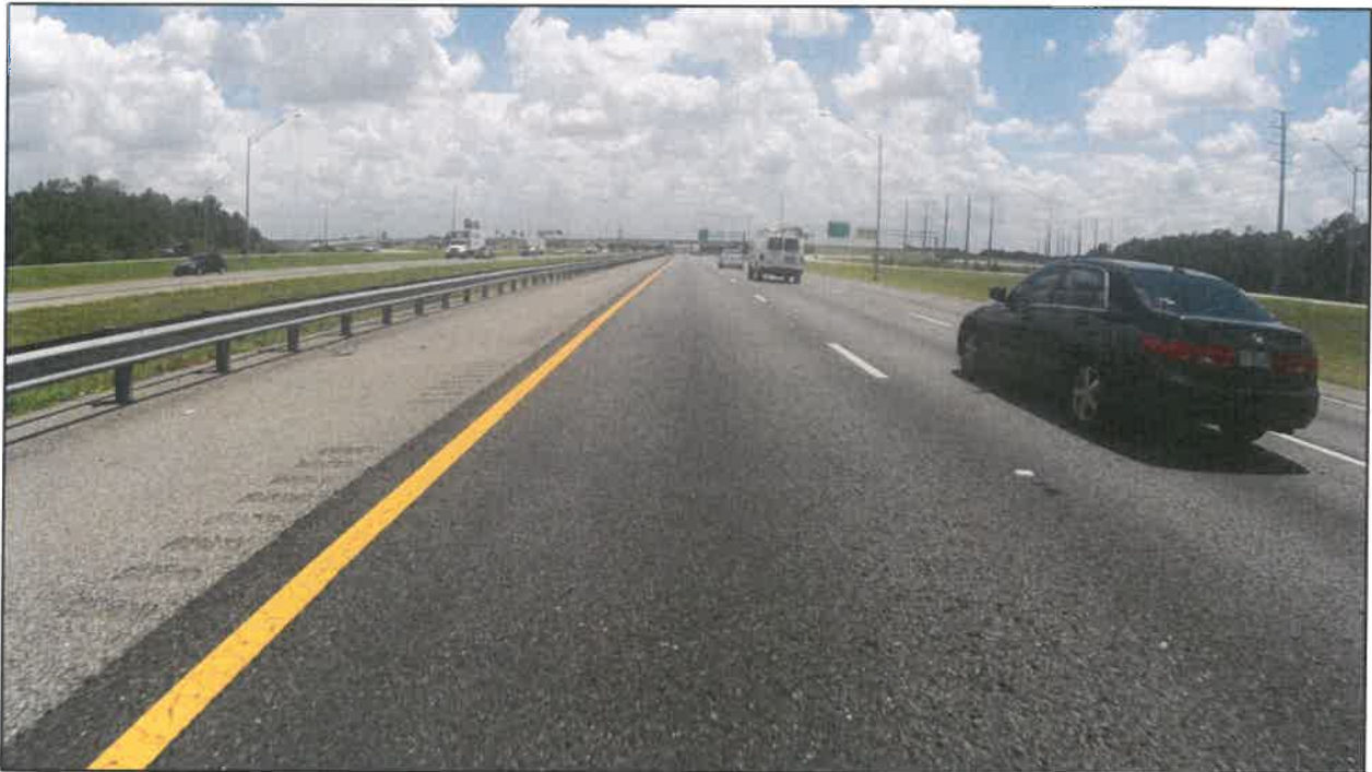
Photo 11: I-4 westbound near MP 4.731. This is a view of the westbound inside paved shoulder. It is in fair to good condition with few if any distresses.
