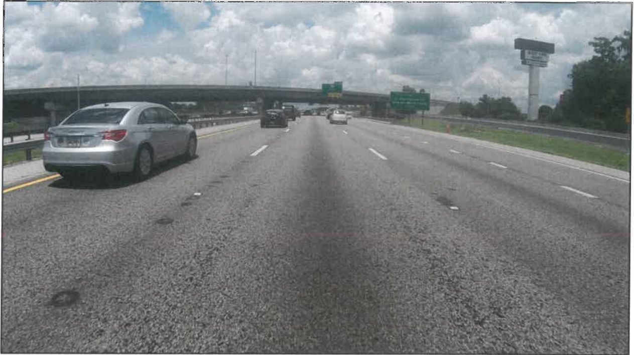
Photo 7: I-4 eastbound near MP 7.611. This photo shows an example of the pop-outs and wear in the wheelpaths in the R2 lane of the FC-5 friction course within the project limits.
