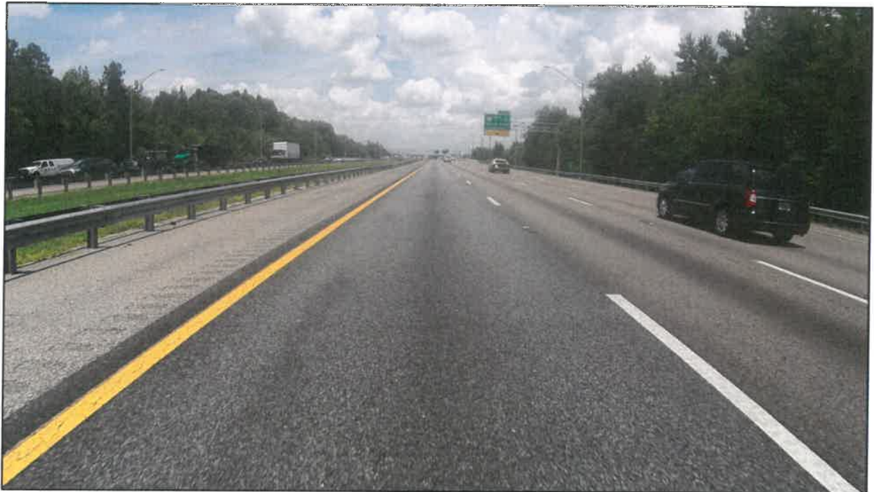
Photo 2: I-4 eastbound near MP 3.346. The inside paved shoulder is in fair to good condition and can be considered an exception to any rehabilitation prior to widening or reconstruction of the roadway.
