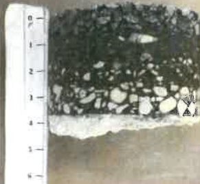
Core #100 500' West of Gore to I-4 EB & WB on SR 530 EB, RAMP
