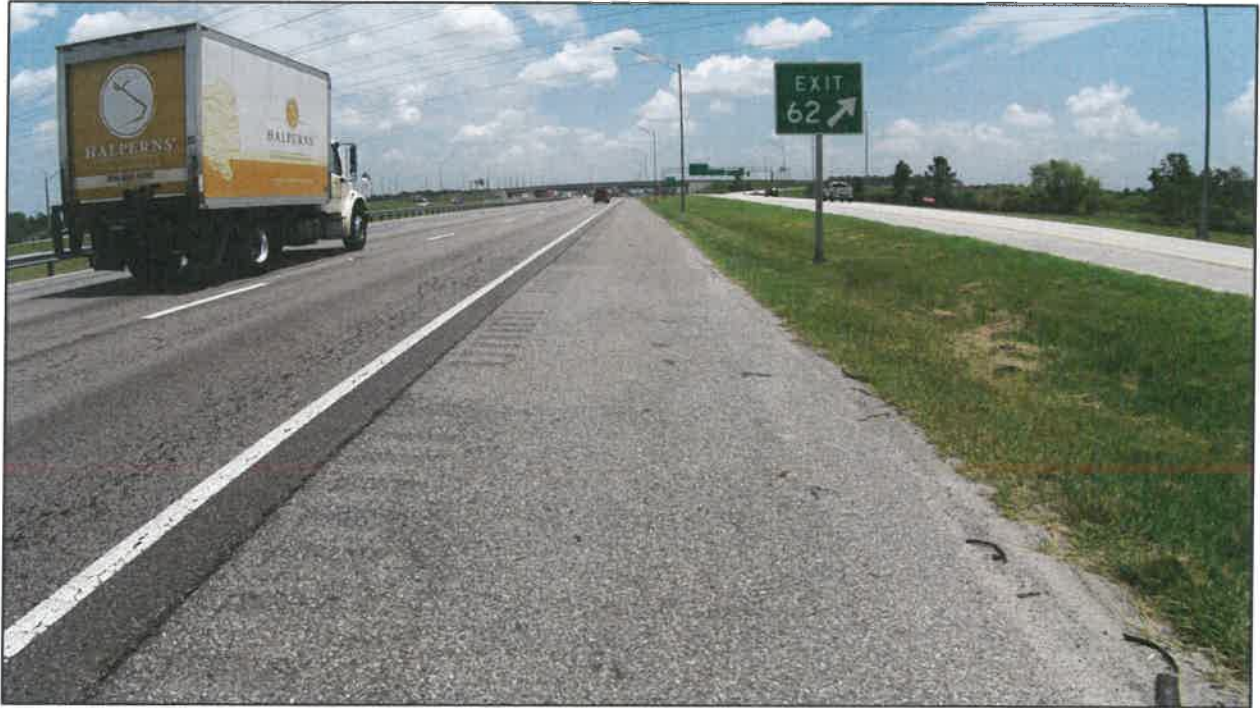
Photo 3: I-4 eastbound near MP 3.851. The eastbound outside paved shoulder is in fair condition, and can be considered an exception to any rehabilitation prior to the widening or reconstruction of the roadway.
