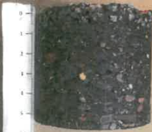
Core #105 Under SR 530 Overpass on I-4 EB to SR 530 WB, RAMP
