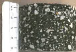
Core #97 1500' West of Bridge over I-4 on Osceola Pkwy EB, R4
