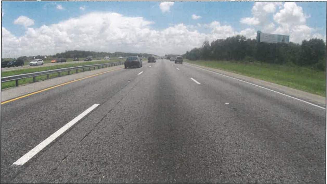
Photo 8: I-4 westbound near MP 0.705. The L2 has light pop-outs and minor tire rim gouging in the wheelpaths.
