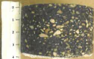
Core #84 1000' West of I-4 Overpass on CR 532, R2
