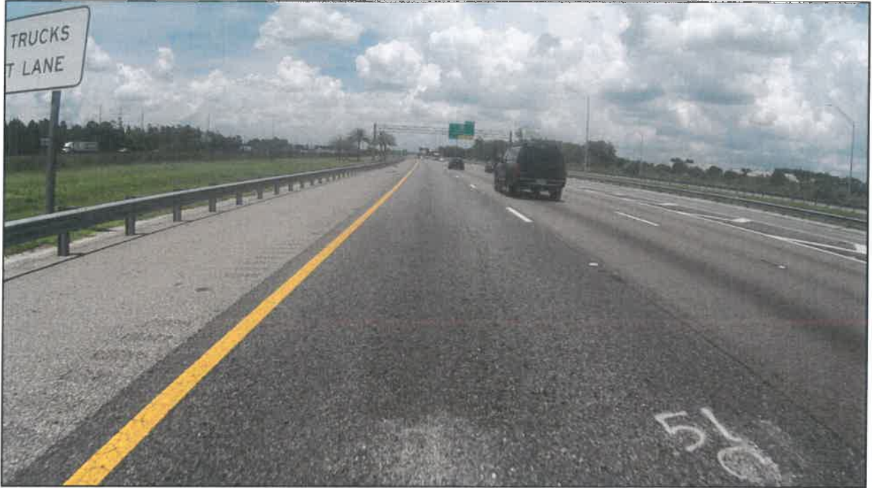
Photo 5: I-4 eastbound near MP 5.250. This is the location of Core 51, taken in the R1 lane. It is located in a lane of widening constructed in 2006 during project FPN 242523-1-52-01.
