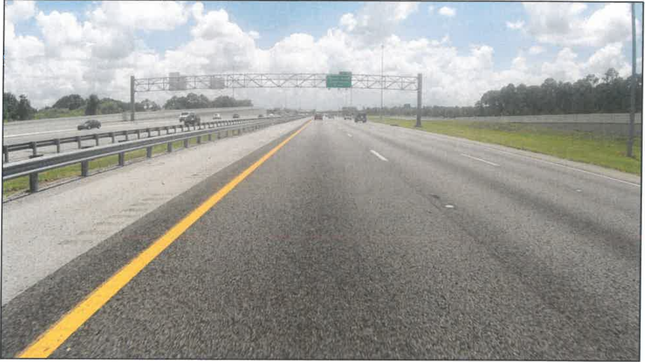
Photo 14: I-4 westbound near MP 7.275. A view of the fair condition of the L1 lane at this location.
