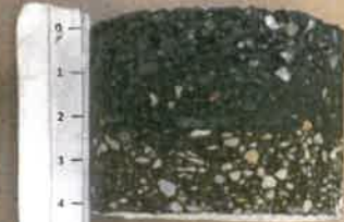
Core #104 500' South of Bridge over I-4 on SR 417 SB to I-4 WB, RAMP
