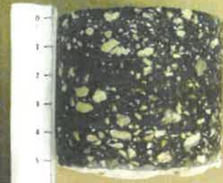
Core #83 530' West of I-4 Overpass on CR 532, R1
