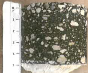
Core #93 Along loop ramp from I-4 WB to Osceola Pkwy EB, RAMP
