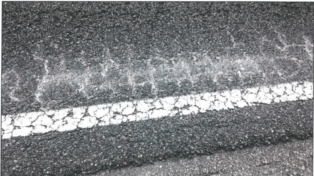
Photo 13: I-4 westbound near MP 4.960. This is a close-up of the limerock pumping shown in Photo 12. This does indicate that the structural and friction courses are permeable to water infiltration.
