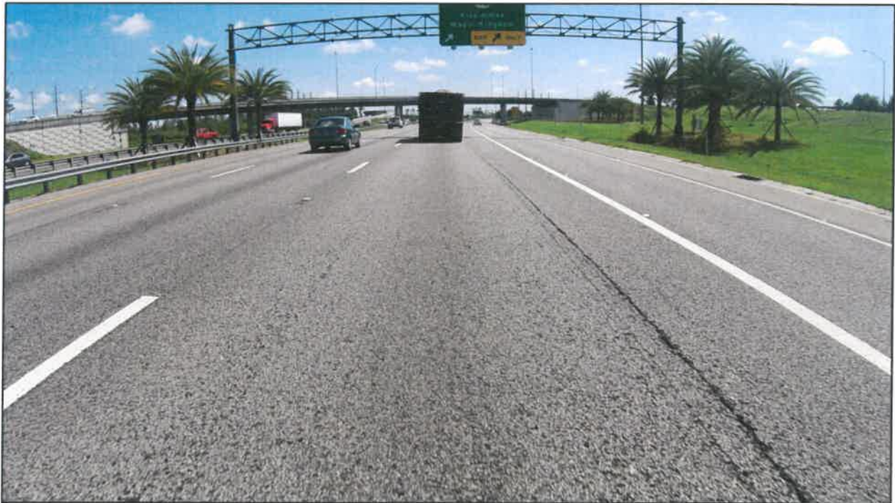
Photo 6: I-4 eastbound near MP 5.901. This photo shows a continuous longitudinal crack that is the separation between the original roadway (the R3 Lane) and an auxiliary lane to the right (the R4 lane) constructed later. The R4 lane has an Asphalt Base Course, while the original roadway has a Limerock base.
