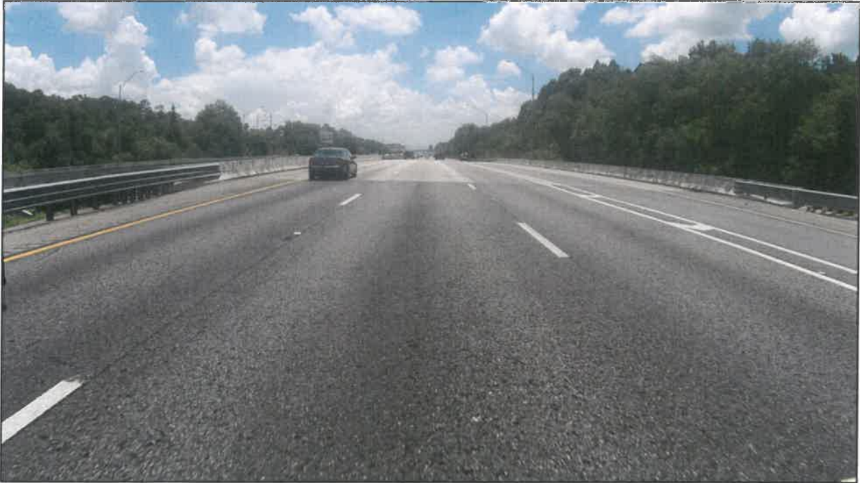
Photo 9: I-4 westbound near MP 3.580. Although the three bridge locations in the eastbound lanes have an asphalt overlay of the bridge deck, none of the westbound spans have one.
