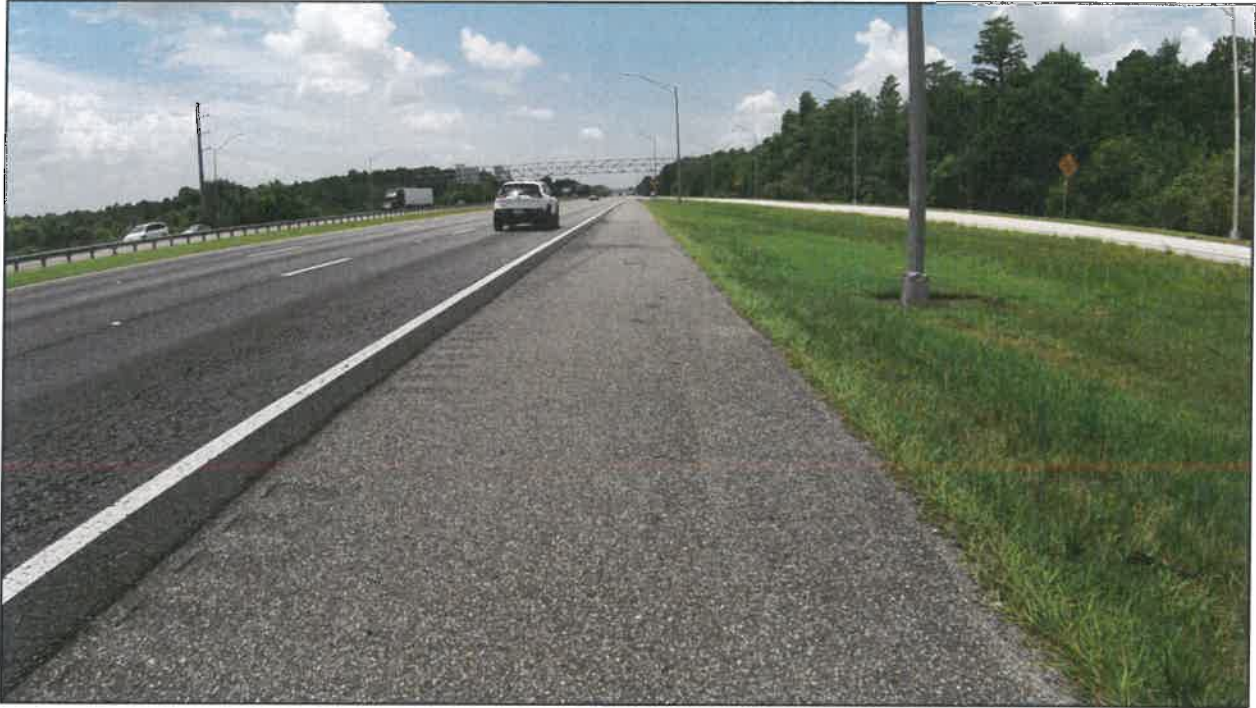
Photo 10: I-4 westbound near MP 3.845. This is a view of the westbound outside paved shoulder. With the exception of a couple of burn scars where there had been vehicle fires, there are no distresses.
