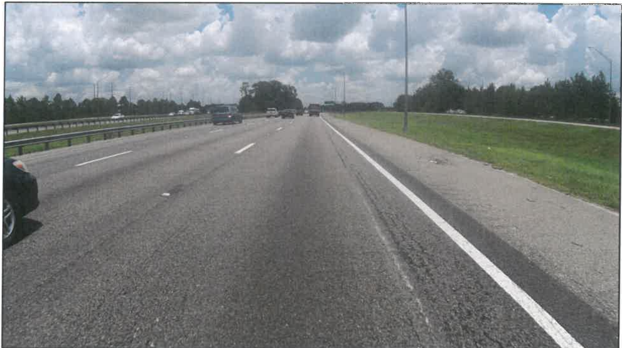
Photo 4: I-4 eastbound near MP 4.971. This is one of the locations where limerock pumping is occurring in both the eastbound and westbound outside travel lanes between MP 2.045 and MP 5.145 (MM 63). This is at the World Drive interchange.
